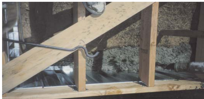
Hang ANCHORPANEL from perimeter, so that panel bottoms are at the middle of a footing trench. Place concrete in the trench.
